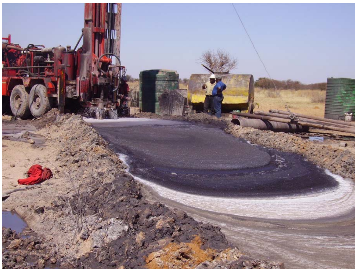
Figure 3-1: Typical borehole drilling in progress and its byproducts
