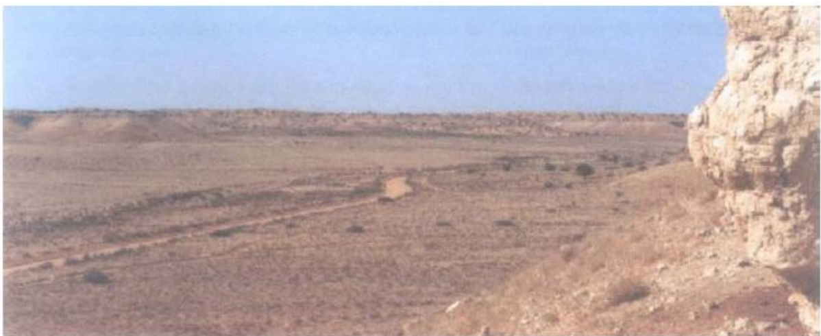
Figure 13: Gravel road to be upgraded in Molopo River Valley at Hoekrans.
